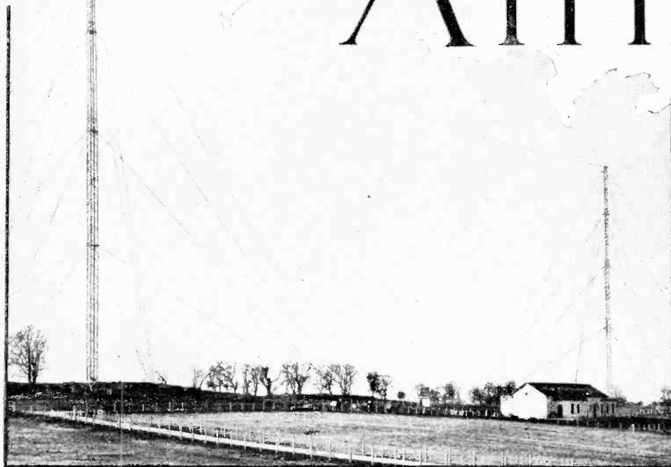
High power alone does not account for the excellence of the Athlone transmissions. The station is situated on an ideal site 300 feet above sea level, and the masts are 330 feet high.
